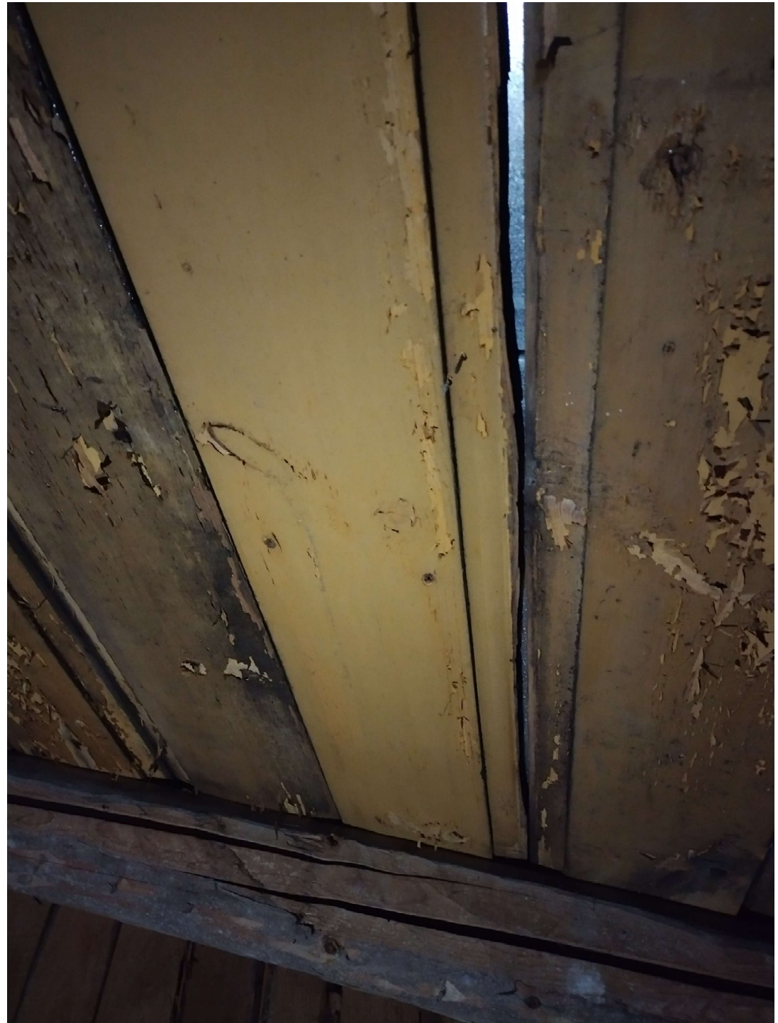
MARELA, OLD RAUMA Detail in the attic
