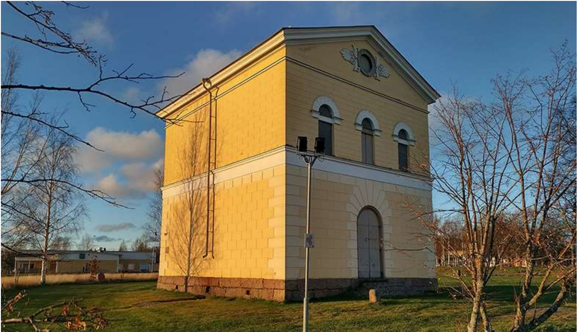
LAVILA MANSION ANNEX – grain storage
